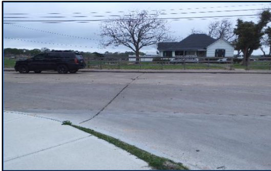
Corner 4 No Ramp (4z)
