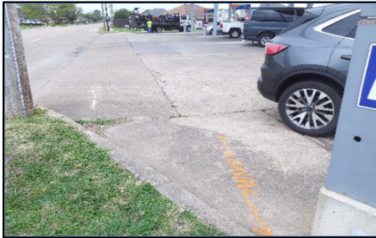
Corner 1 No Ramp (12)
